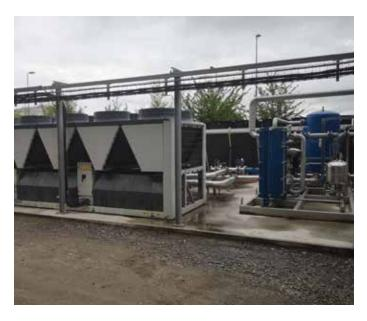
thereby minimizing the average energy consumption during the sugar campaign. When the ambient air is below 15°C, only the dry cooler will operate, while the dry cooler and chiller will work from 15 C to 28°C. At temperatures above 28°C, only the chiller will operate (see Graph 1). With this combination, the cooling water will always be at a consistent 18°C.
