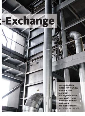
sand quality. By reducing the generation of dust and mitigating the chance of dust egress, moving bed heat exchangers also lessen the loads on existing baghouses and dust collectors.
