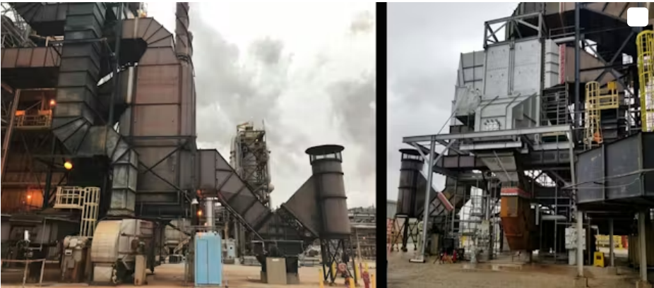
Figure 6: (Left) An existing DEKA air preheater with structure and ducting. (Right) A retrofit HPHE air preheater with adaptive transition pieces.
