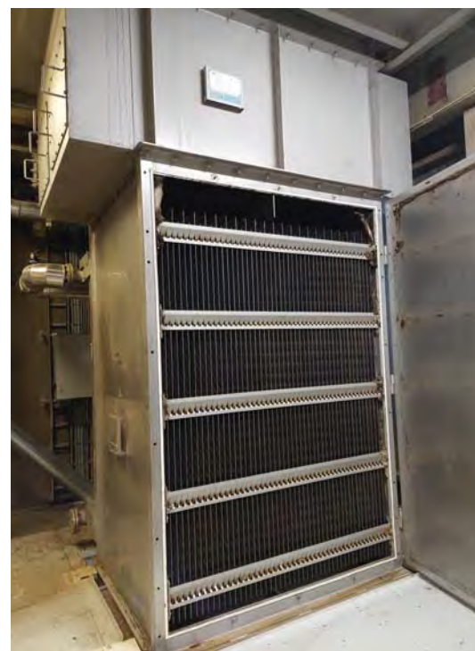
➤ Meal pre-heater showing the stainless-steel pillow plates. Courtesy of Solex Thermal Science.
