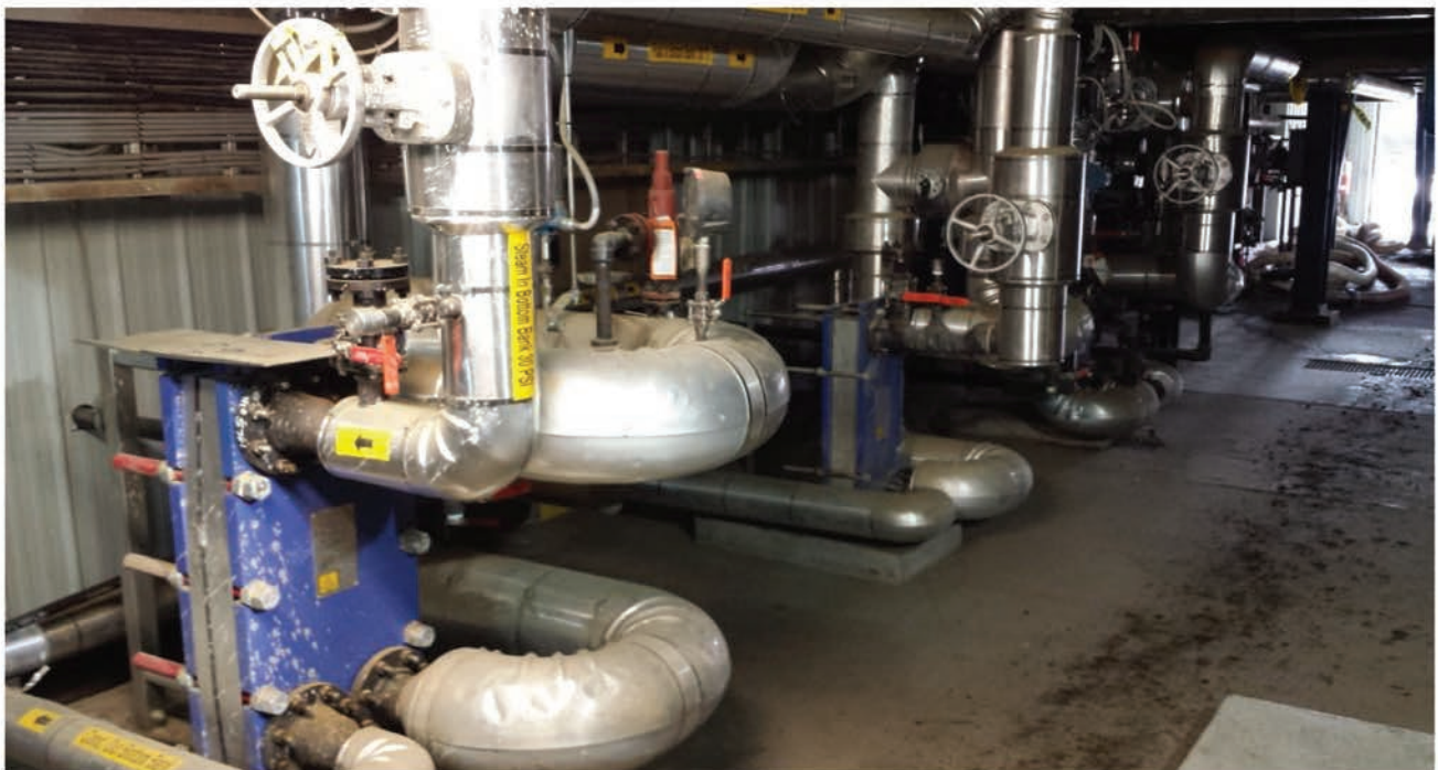
In an oilseeds installation, three heat recovery loops are used to recover waste heat and recirculate it to preheat the seeds.
