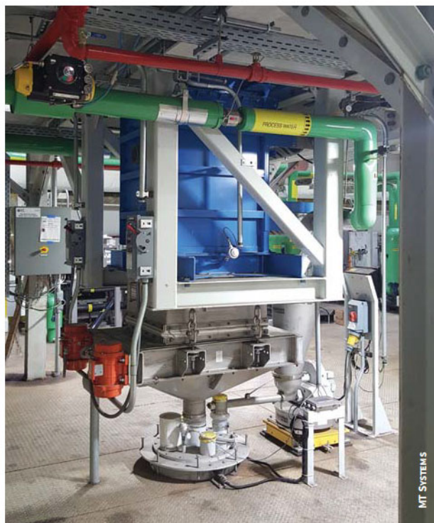
The capacity of the Solex coolers is typically designed to be 15 to 30 minutes of supply.
