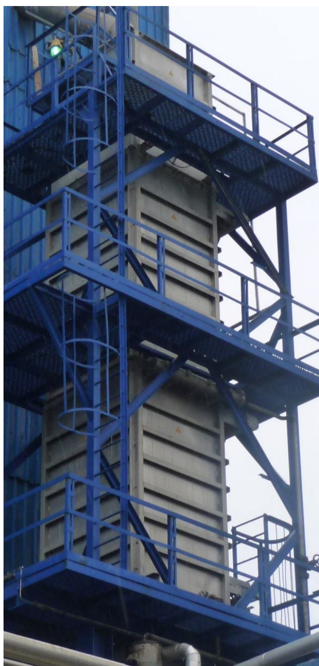
Figure 2. Solex heat exchanger installation.
